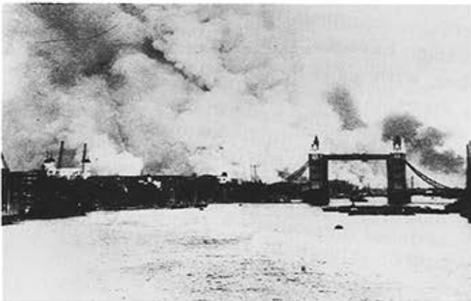
The Blitz - The Docks of London Burning viewed from Tower Bridge.
